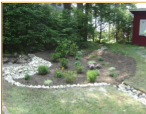
*Rain Garden* - pervious detention basin designed to store stormwater during a rain event and allow it to infiltrate. Typically a trench directs water into the rain garden. Water tolerant plants are put in to uptake additional water and absorb excess nutrients.
