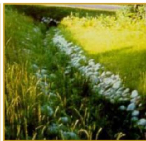
*Ditching* - Once water is directed off the road, it should flow into a pervious ditch to allow it to infiltrate. There are various methods such as vegetation and check dams which can be used to slow stormwater down in a ditch.
