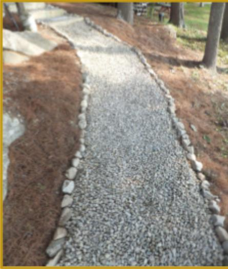
*Infiltration Path* - a trench filled with crushed stone that traps stormwater. Can replace dirt paths susceptible to runoff.
